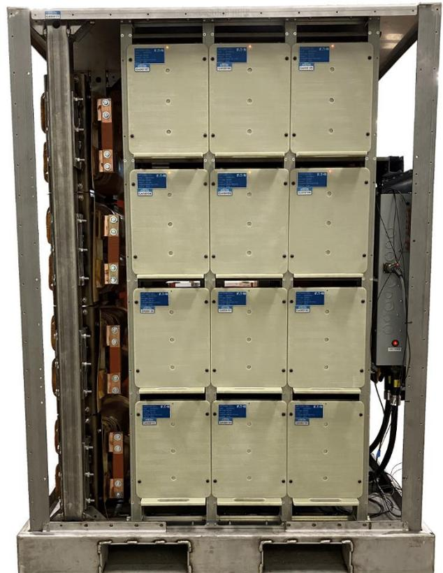
**Fig. 4:** Modular units on the front of the prototype breaker
