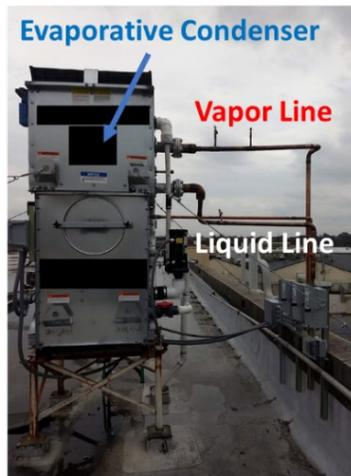
**Figure 3. An evaporative condenser integrated with the loop thermosyphon. The condenser is located on the rooftop of Burle business park where ACT is located.**
