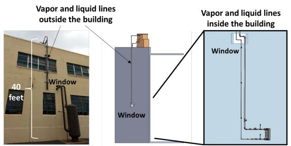
Figure 5. Left: Picture of the vapor and liquid lines outside the building. Middle: 3D drawing of the test setup. Right: Vapor and liquid lines inside the building.
