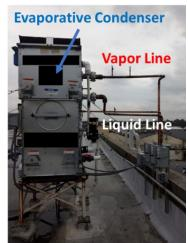
Figure 3. An evaporative condenser integrated with the loop thermosyphon. The condenser is located on the rooftop of Burle business park where ACT is located.
